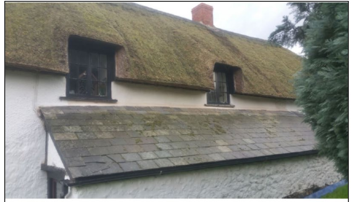
Image B: Existing brick chimney to be raised by approximately 3 x courses of bricks
