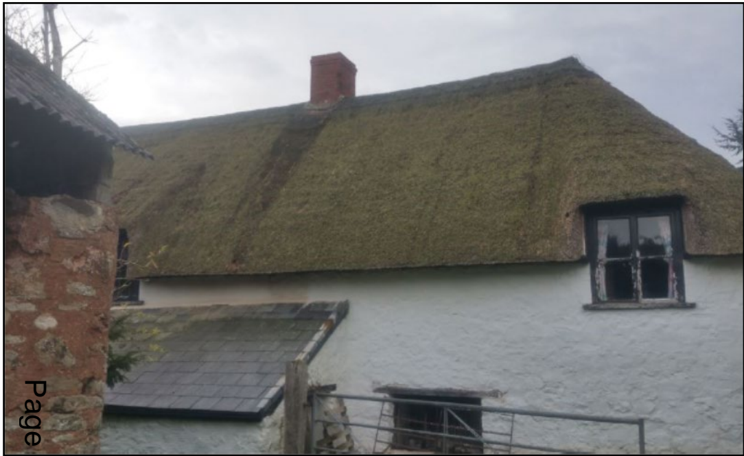
Image A: Existing brick chimney to be raised by approximately 3 x courses of bricks
